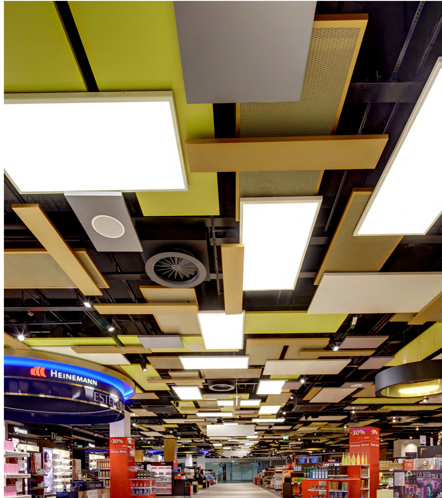
HEINEMANN SHOPS, VIENNA, AUSTRIA
